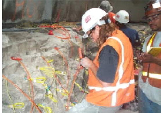
**Figure 1 – Blasting very close to a concrete caisson**
