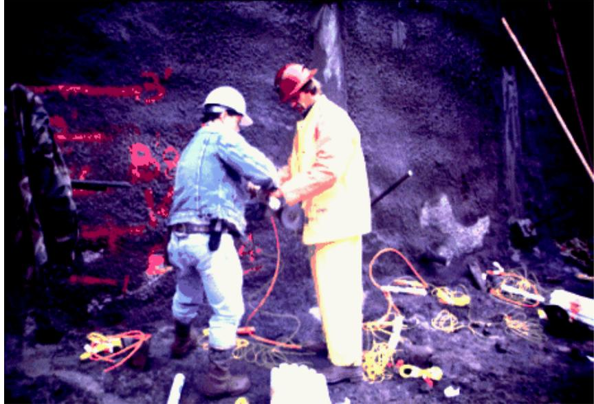
**Figure 2 – Using very light charges to prevent damage to soldier piles and to produce smooth walls.**
